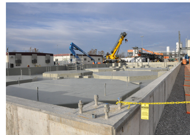
The Super Critical Water Oxidation (SCWO) tank farm pads are set, coated and tanks are currently being erected in this area
