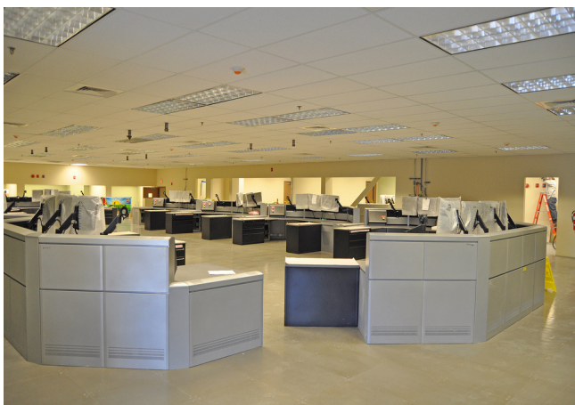
Consoles in the control and support building allow operators the ability to remotely control and monitor the chemical demilitarization equipment
