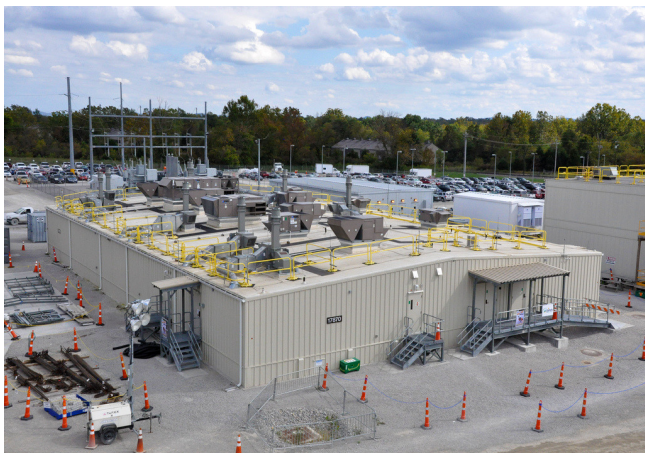
Chemical agent destruction will be verified in the laboratory building
