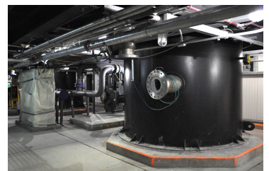
The Thermal Oxidizer (TOX) will treat gaseous byproducts of the chemical demilitarization process including PCBs
