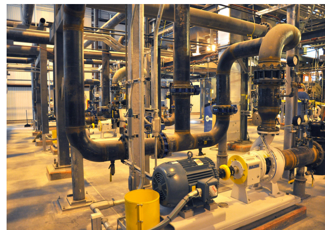
Massive runs of piping in the utility building (UB) distribute various process chemicals, water, and steam throughout the BGCAPP
