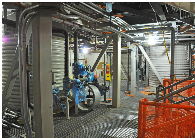
The energetic neutralization reactors (ENR) treat the energetic hydrolysate from the energetic batch hydrolyzer (EBH)
